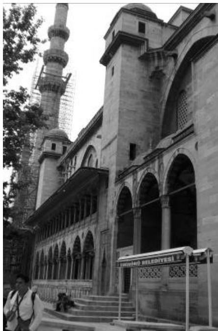
Figure 3 (left): View of right side wall according to the main entrance axis, with columns connected with iron bars; (photo by Yesim Kamile Aktuglu on 7 th of June 2008)
